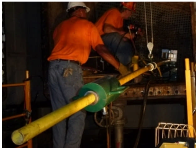
Gin Pole Connected to an Electric Hoist
